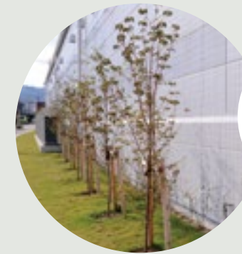
A green curtain installed on the exterior wall of a store
