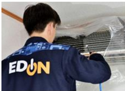
Air conditioner cleaning
