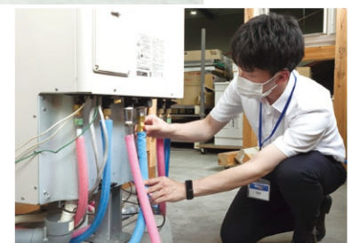
EcoCute installation training (inside the Toyota Service Center)
