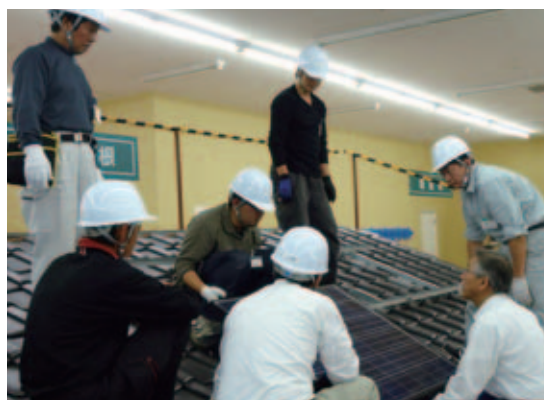
Construction work training for home solar power generation system
