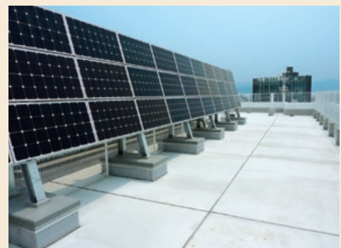
Solar Power Generation System installed on roof of EDION Hiroshima Main Store
