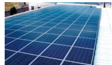
Industrial use solar power generation system
