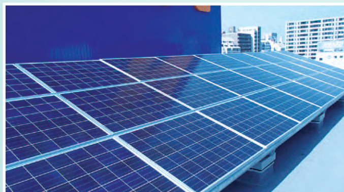
Solar power generation systems installed on the roof of the EDION Nagoya Main store
