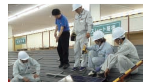
Construction work training for home solar power generation system
