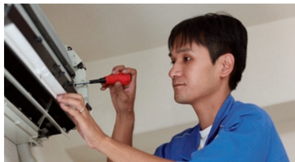
Repair service at customer's home
