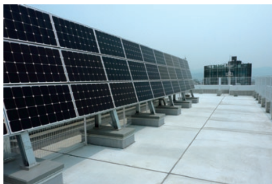
Solar Power Panels Installed on Roof of DEODEO's Main Store Annex
